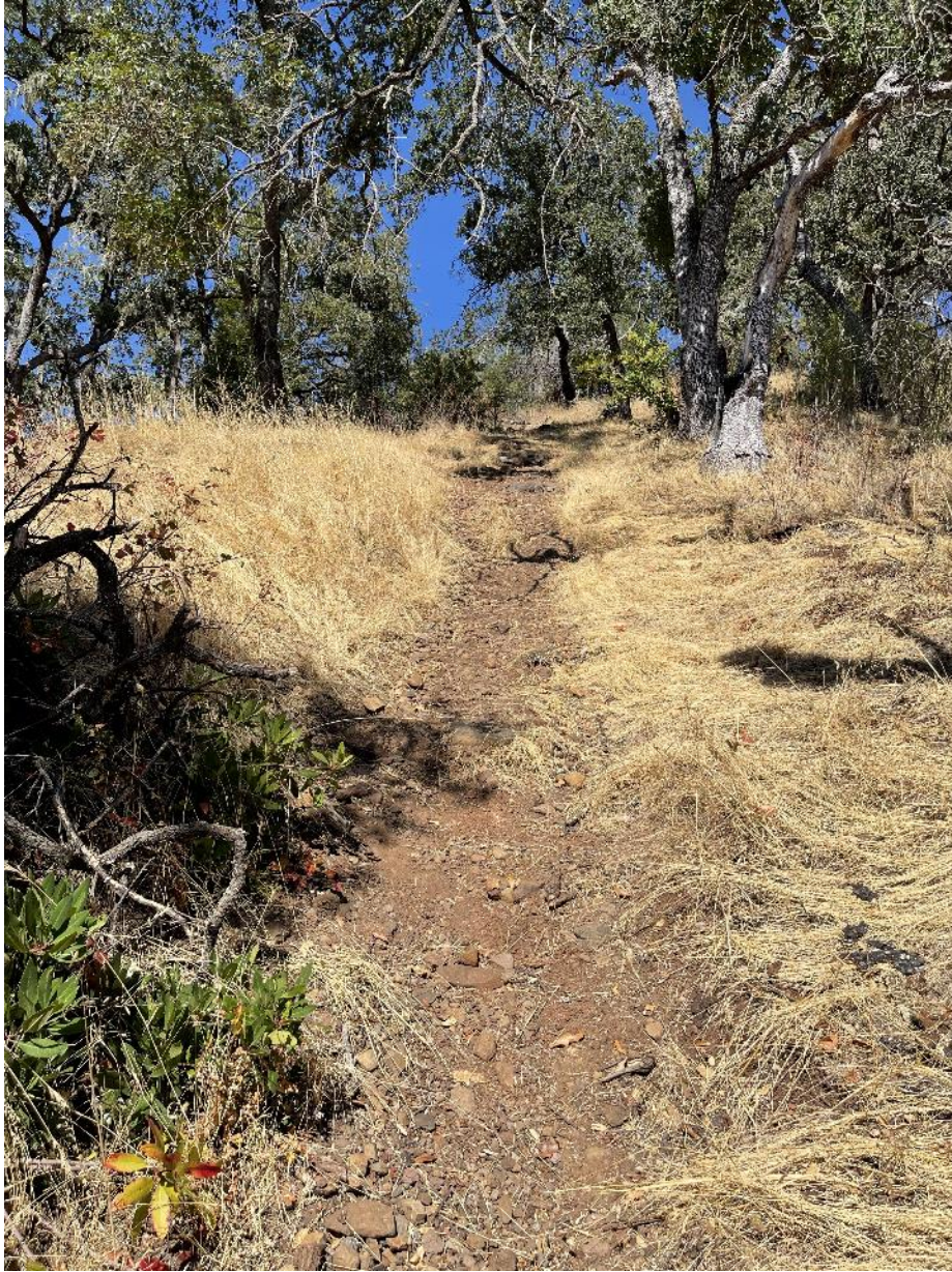
Figure 51: Chronic Erosion Site #8, Impossibly steep, former fire service road northwest of the Lake Suttonfield dam with rutting evident. This trail is still being used by hikers and mountain bikers transiting south from the Sonoma Valley Regional Park trails with moderate safety risk of doing so.
