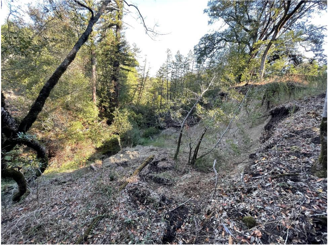
Figure 43: Chronic Erosion Site #3 at confluence of Roulette and Asbury Creeks. Quarry scale amounts of fine sediment have been eroding to Asbury and Sonoma Creeks from this location for the past two decades.
