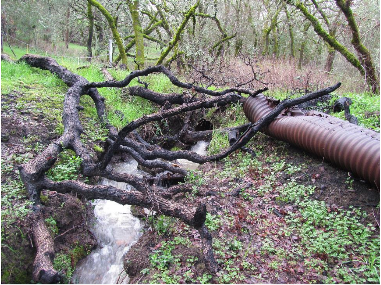
Figure 38: Chronic Erosion Site #1, Culvert-related gully erosion just north of developed campus at bottom of Corridor Creek South.
