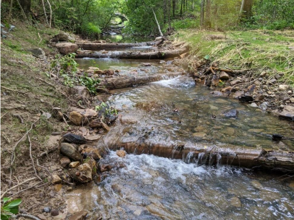
Figure 33: Water Retention Opportunity #9, Example of “Stage Zero” creek restoration involving large wood “aquatard” structures embedded into the stream banks.
