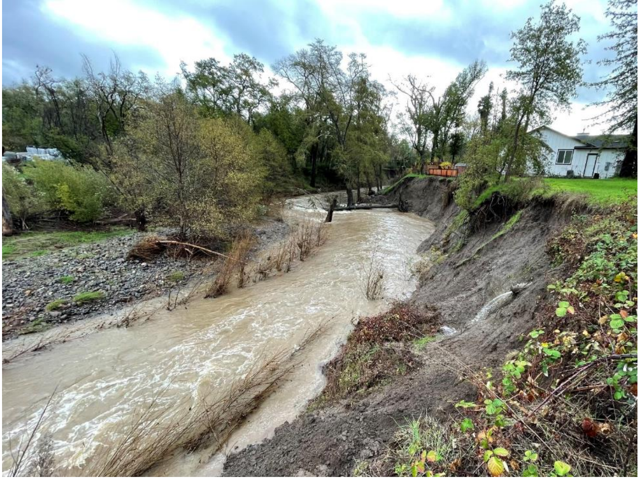
Figure 41: Chronic Erosion Site #2, Bank failure on Sonoma Creek at downstream end of SDC reach. Nearby house is threatened.
