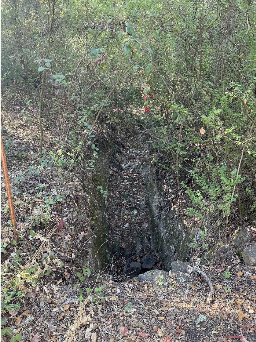
Figure 13: Constructed channel leading from Fern Lake overflow spillway to Roulette Creek via Great Meadow. Shown here is the place where the channel crosses the primary service road leading to the diversion point on Asbury Creek.
