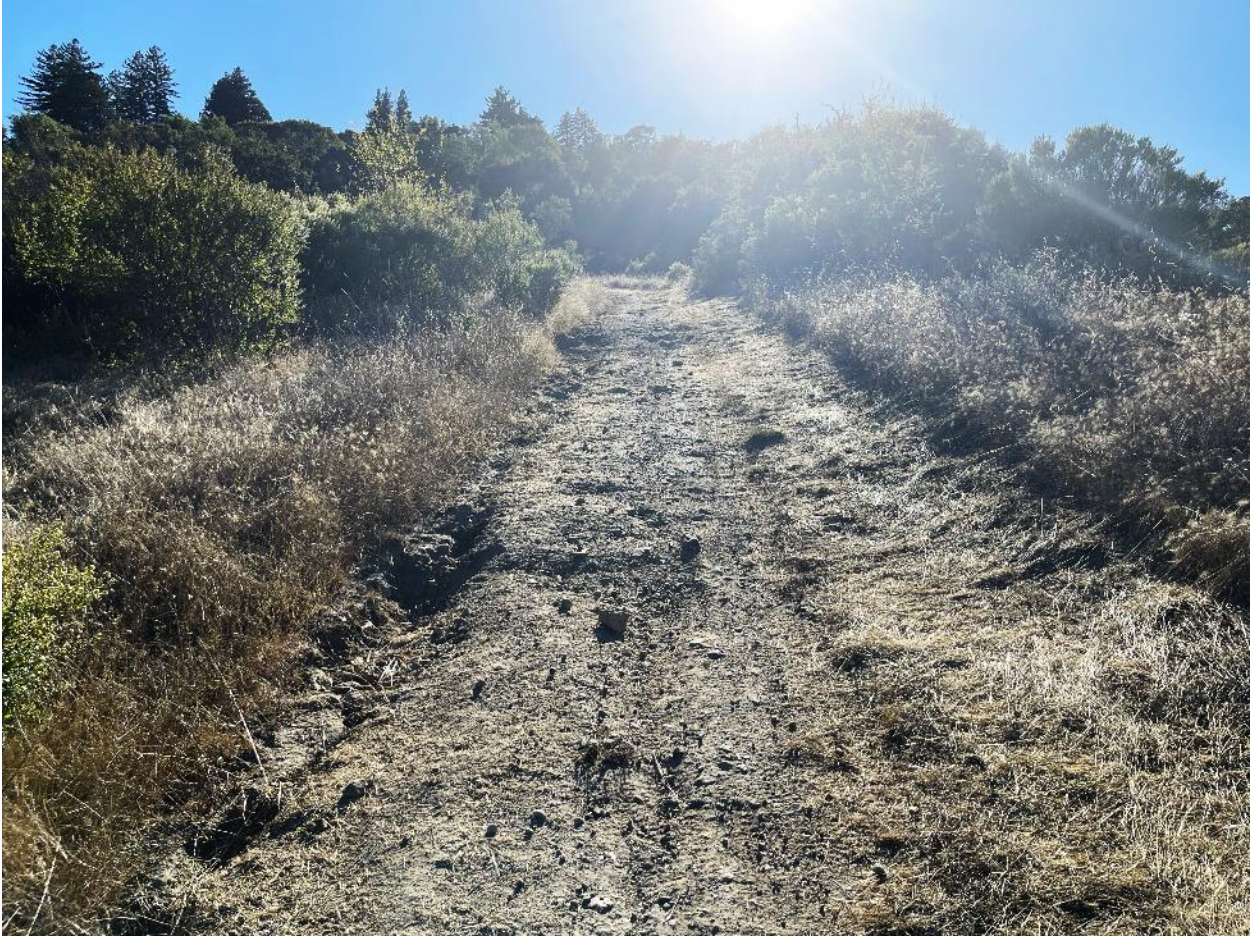
Figure 48: Chronic Erosion Site #6, Rill and gully erosion on a steep section of a primary fire service road running through the western SDC open space within the Sonoma Valley Wildlife Corridor. A seep occurs at the top of the steep section and hikers, bikers and horseback riders using this adobe laden route during the wet season continually promote rill and gully erosion here.
