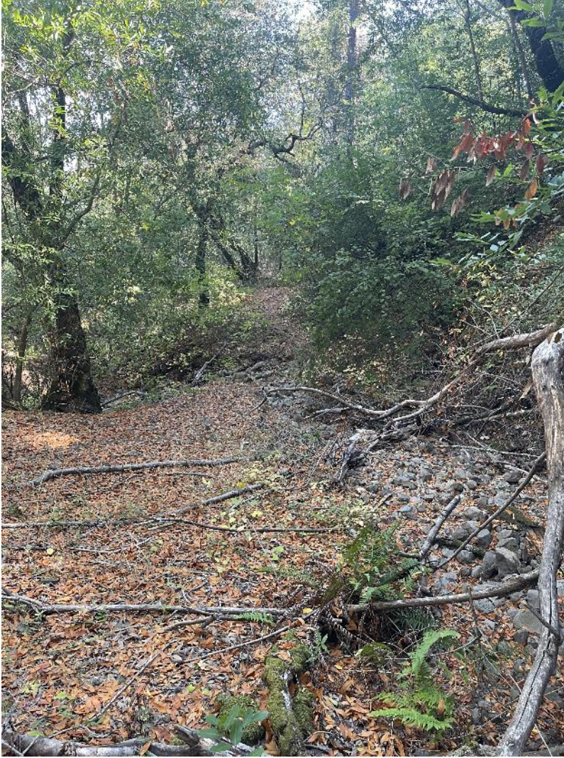
Figure 12. Water Retention Opportunity #3, road and drainage erosion below sluice canyon.
