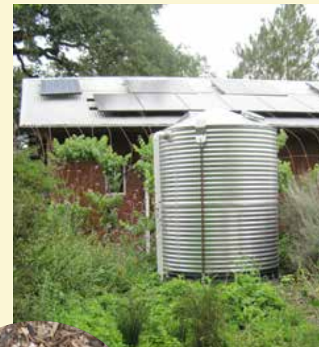
Above: A 20- x 30-foot roof with a roof water catchment system saves 11,000 gallons a year with the annual rainfall of Sonoma Valley.
