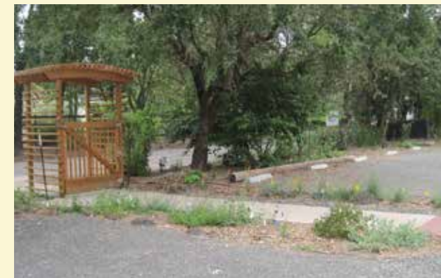
Above: The gravel parking lot and swales capture and filter stormwater and recharge groundwater.
